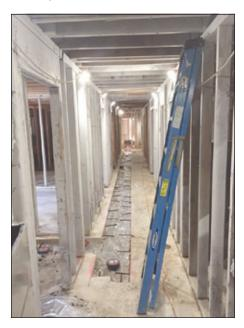
We are happy to report that progress is being made in restoring our building. All our architectural plans have now been approved by the City of Wheaton. The roof has been reconstructed, rough plumbing has been done, the HVAC system is being installed, doorways are being built, windows are being replaced, and the interior framing is underway. We are anticipating that the building will be ready for occupancy by summer's end.
